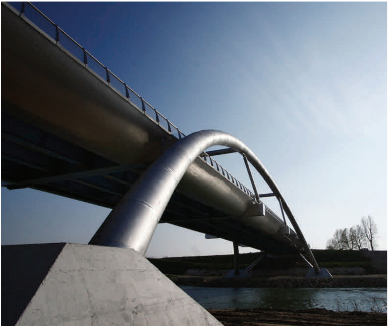
Bridge , made of duplex stainless steel, crosses a river in Italy.
