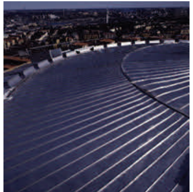
Roof made of stainless steel
